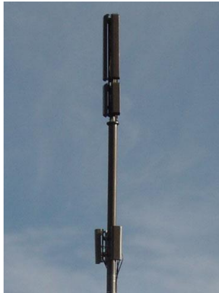
Flush Mount Install
